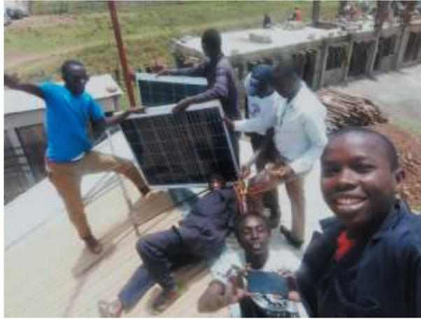
Figure 13. LED module 1 students and teachers at Tumaini installing the final design solution (solar PV system to address lack of reliable power source).
