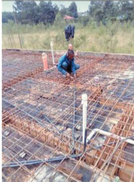
Figure 12. Stellar graduate at a project site installing electrical wiring system for on-going construction.
